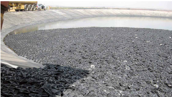
BULK delivery and installation
