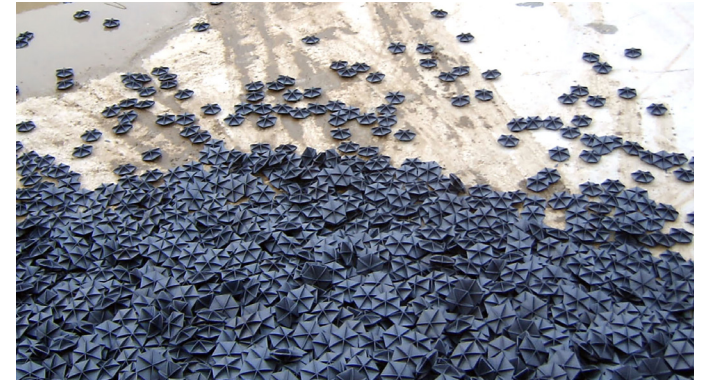
Installation in empty tank, no problem !
