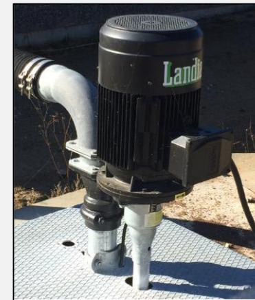
*Landia's long-shaft pumps are installed on the side of a well or a tank so that the lower part of the pump housing is submerged in the manure while the upper part, including the engine, is up in the open*
